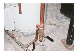
Background- Due to some water heater brands having an anode rod that is combined with the hot water outlet nipple, a question arose in my mind as to whether an anode placed in a chamber exterior to the tank would still provide cathodic protection to the tank. If it were to work it would provide extended water heater life by making it easy to replace the anode rod at periodic intervals.
