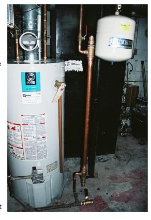
Presently there is no corrosion evident at any bimetal tank connections on the top of the tank and only slight discoloration at the T&P boss. The experiment calls for the inspection of the anode at regular intervals to determine rate of decay and to visually inspect tank connections for corrosion.
